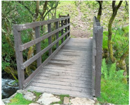
New bridge over Tongue Gill
