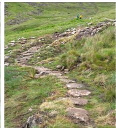
New section of pitched path that avoids the bedrock
