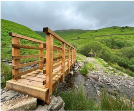
New bridge over Little Tongue Gill
